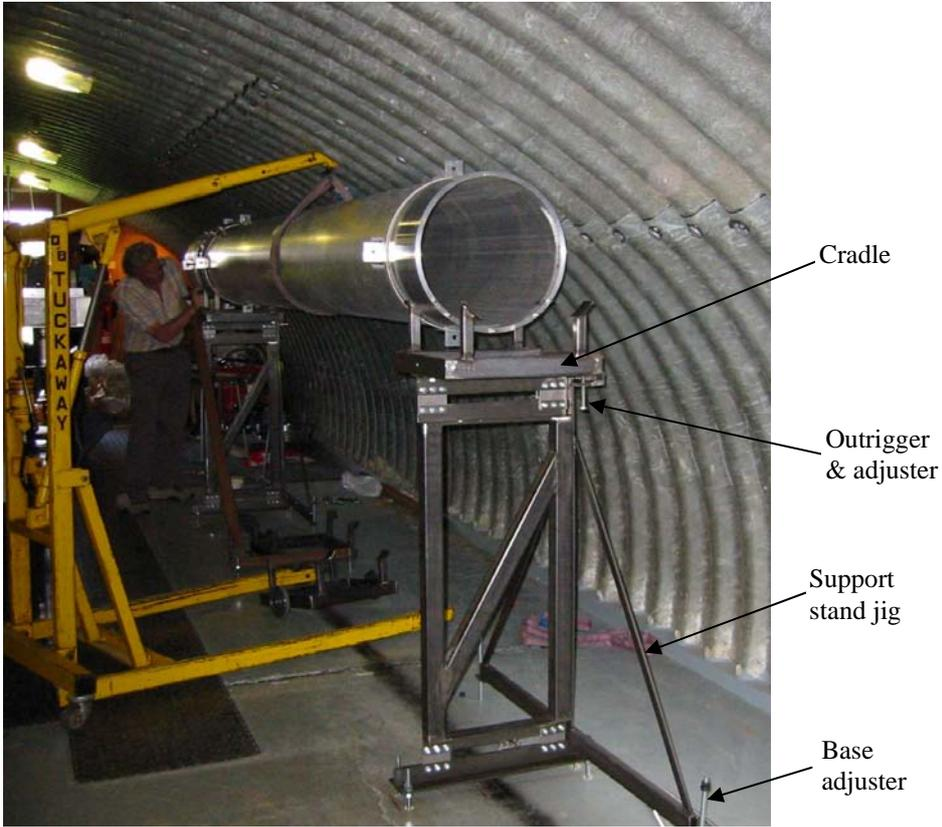
Figure 4 Photograph of a pipe being positioned on a cradle with the support stand jig applied to the support stand to stabilize both the stand and the cradle.
