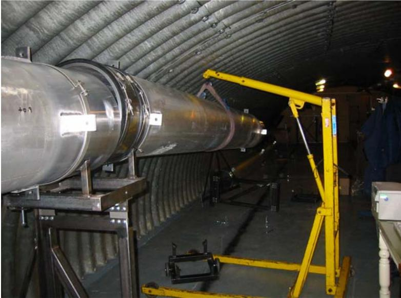
**Figure 7** Lifting a pipe section into place. In this case the seal is on the pipe being fitted. The stand at the other end is not yet erected because maneuverability of the pipe is restricted by ceiling height
